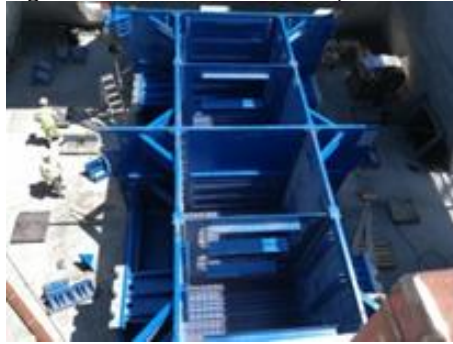
Fig. 1. Internal compartments of the steel box (Structurae, 2020).
