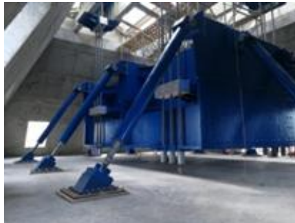
Fig. 2. Cross hydraulic dampers and pendulum cables.
