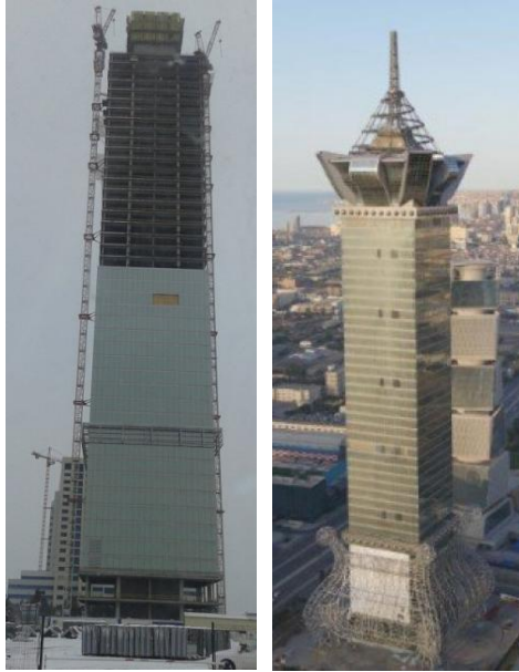
Fig. 4. Views of the IT construction phases (Council on Vertical Urbanism, n.d.)
